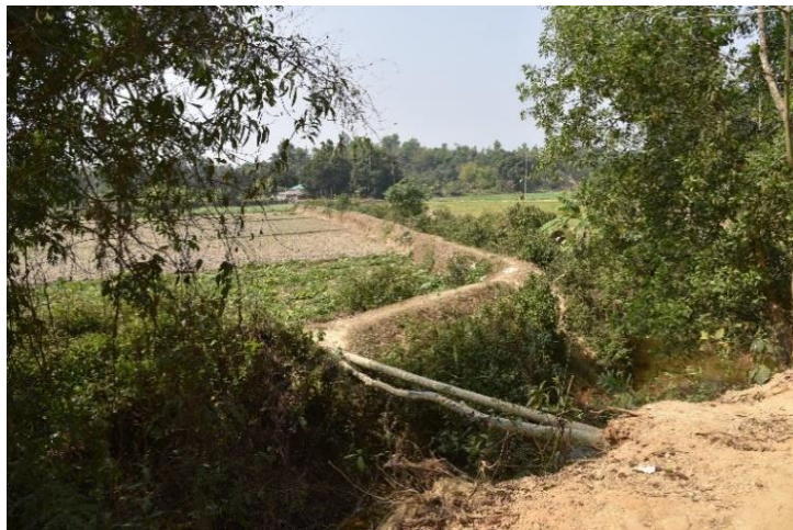
Pre-condition of Hangorghona Bamboo Bridge at Baruapara Village in Rajapalong Union, Ukhiya (Photo: Mahtabul Hakim/UNDP)
